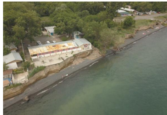
Fig. 4. Results of shoreline erosion at Akshi village (photo by the author, 2019)
