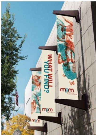
Figure 13. Installing signage using a bracket on the facade
