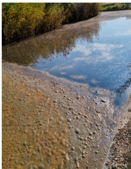
Figure 2. Sludge drying beds of the Astana WTP (photographed by S. Merkýreva, 2022).
